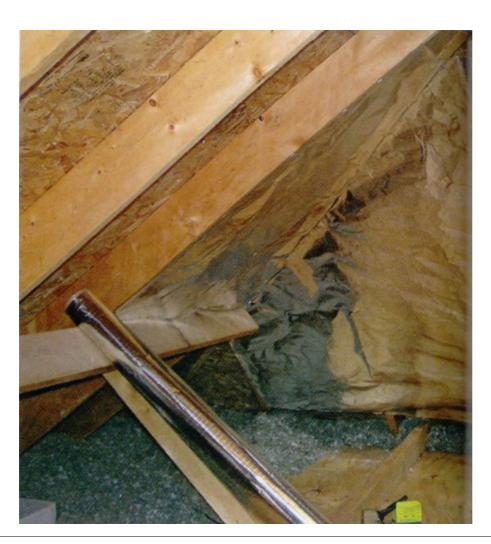
Radiant barrier (the shiny foil-like material attached to the roof rafters) reduces heat gain.
